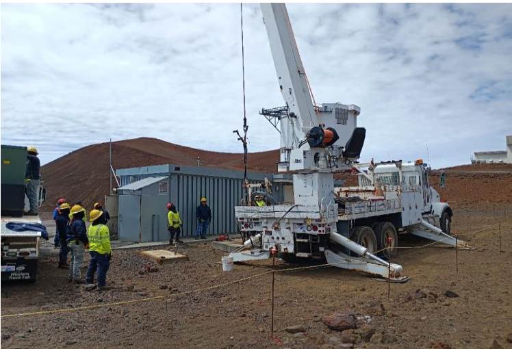
^ 12:34pm - pulling cables from the conduits
