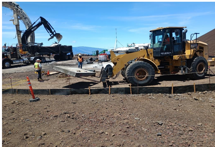
^ 11:07am - relocating concrete transformer pad
