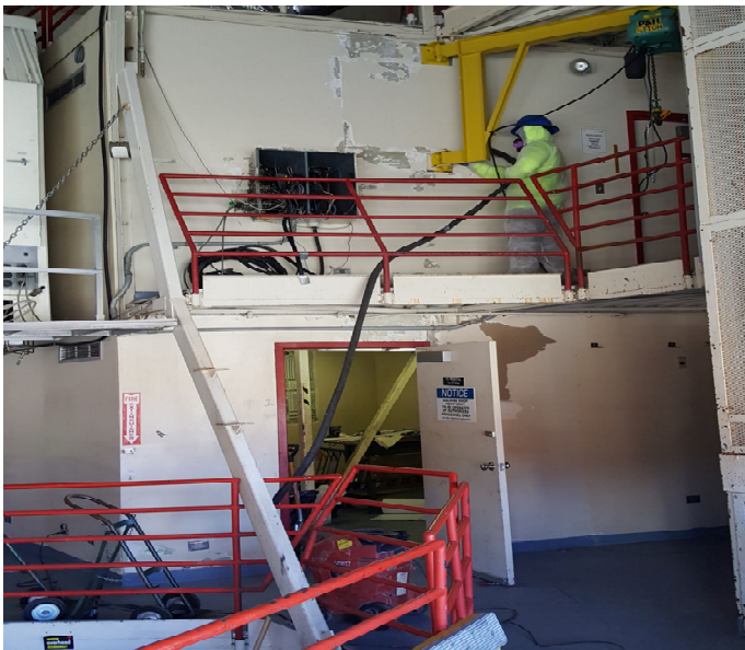
Scraping and Vacuuming Areas of Loose Lead Paint
