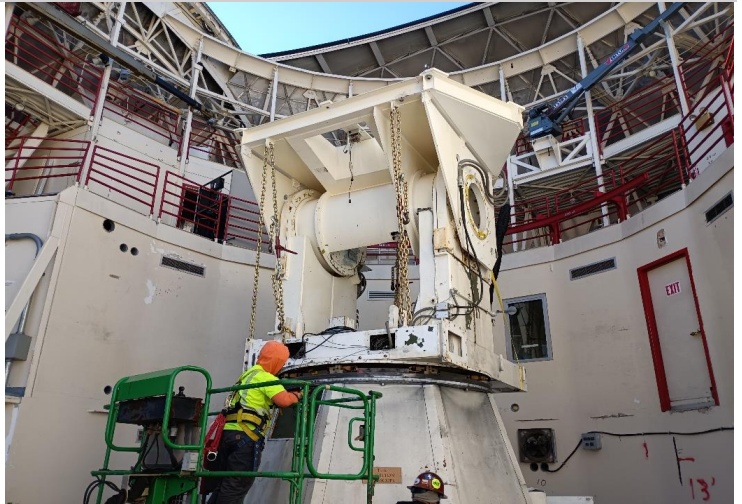
^ 9:17am - continuing prep of elevation assy for removal
