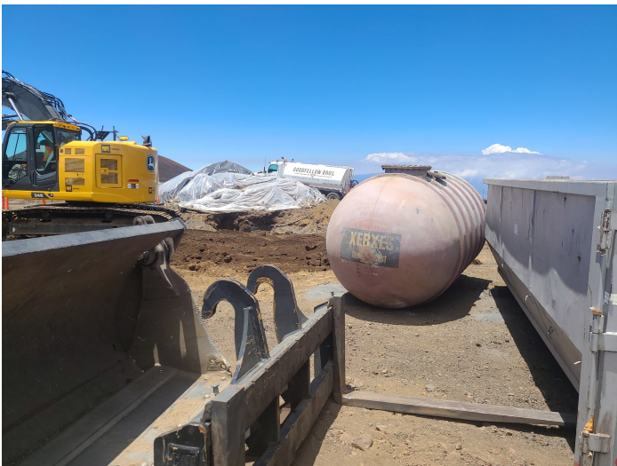
^ Salvaged Underground Fiberglass Water Tank
