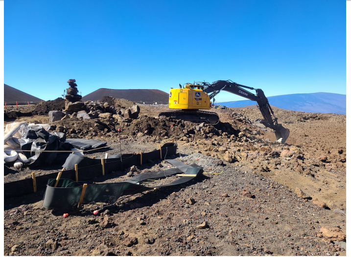
^ Excavating and Stockpiling Stones North Perimeter
