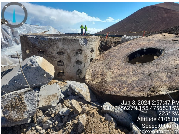
^ Cesspool Precast Ring and Base
