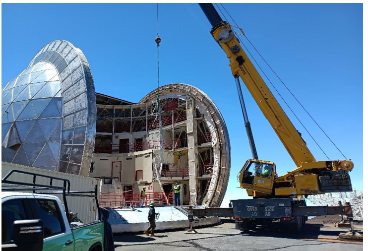
^ 11:15am - removing parabolic truss from dome
