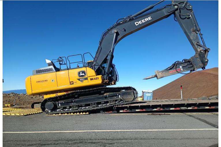
^ 8:08am - loading excavator, pavement protected with mats
