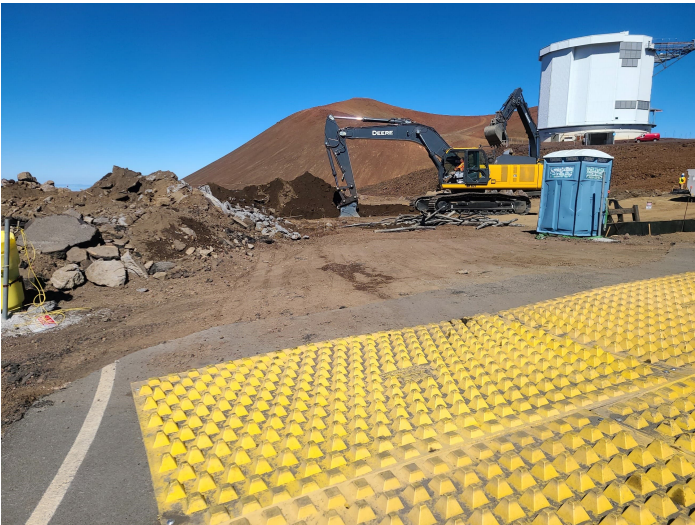
^ Excavating Utility Ducts From CSO Dome to Utility Shed
