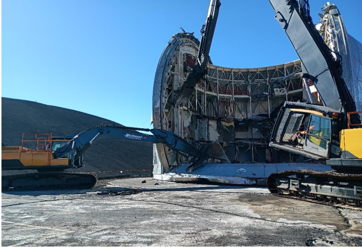
^ 8:25am - housing demo for cylinder removal
