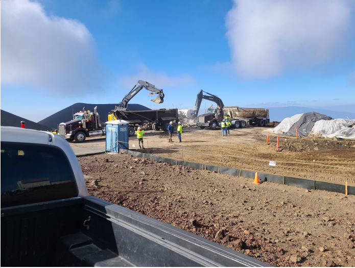
^ CSO Concrete Rubble Loading Deluz Truck
