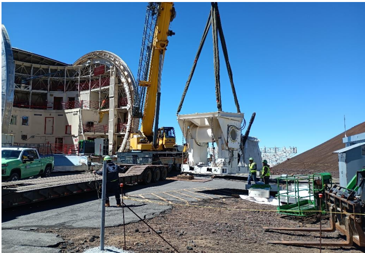
^ 10:37am - elevation assy being moved to lowboy
