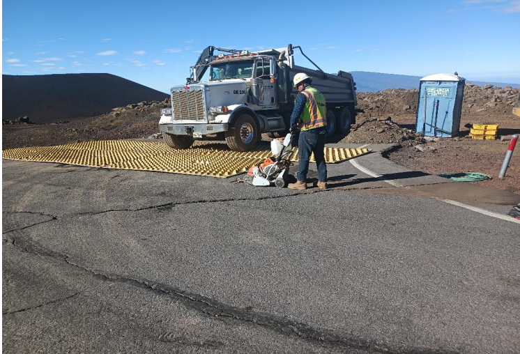
^ 8:18am - sawcutting pavement
