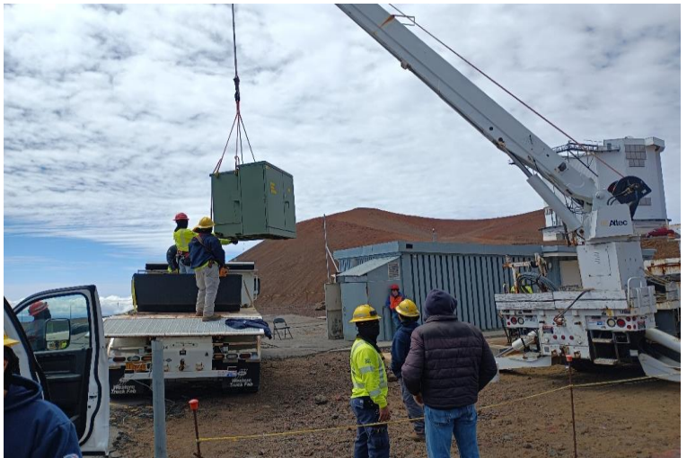
^ 12:31pm - removing transformer from pad to truck
