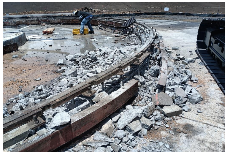
^ 12:52pm - demoed section of rail ring (dust control water visible)
