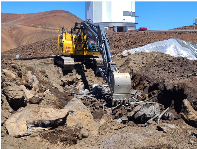
^ Ripping Ducts and Concrete Jacket at Center of CSO
