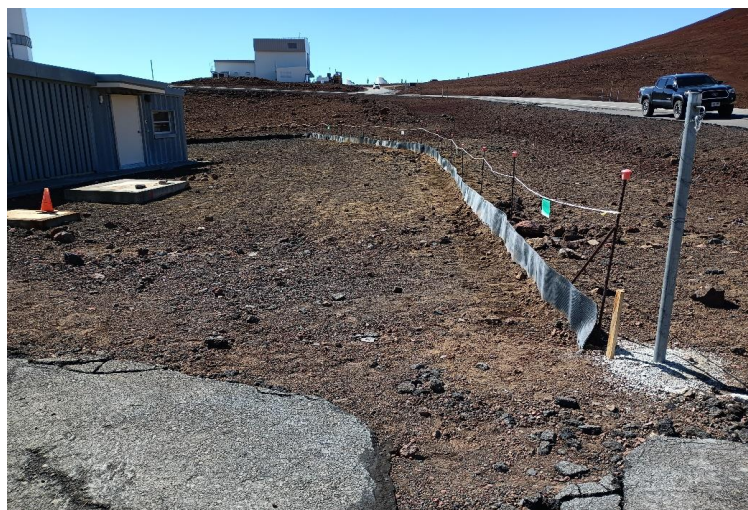
^ 3:09pm - finished silt fence
