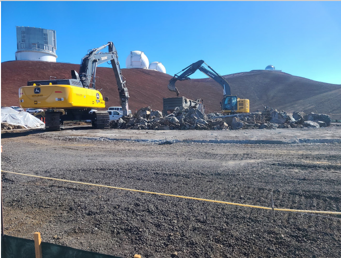
^ CSO Concrete Apron Demo and Loading Deluz Truck
