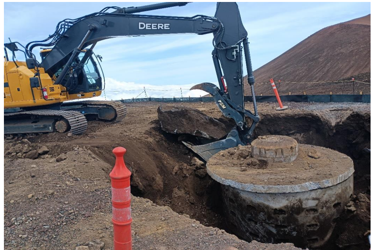
^ 2:22pm - cesspool excavation
