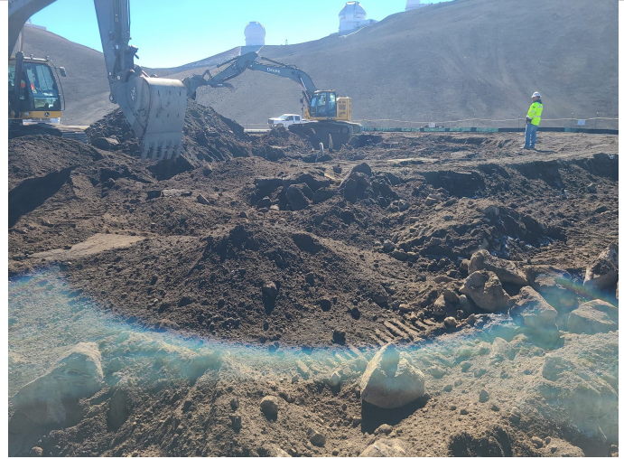
^ Ripping CSO Foundation, Pipes, and Ducts
