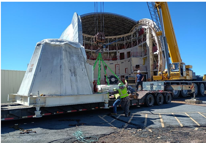
^ 9:45am - counterweight positioned on lowboy
