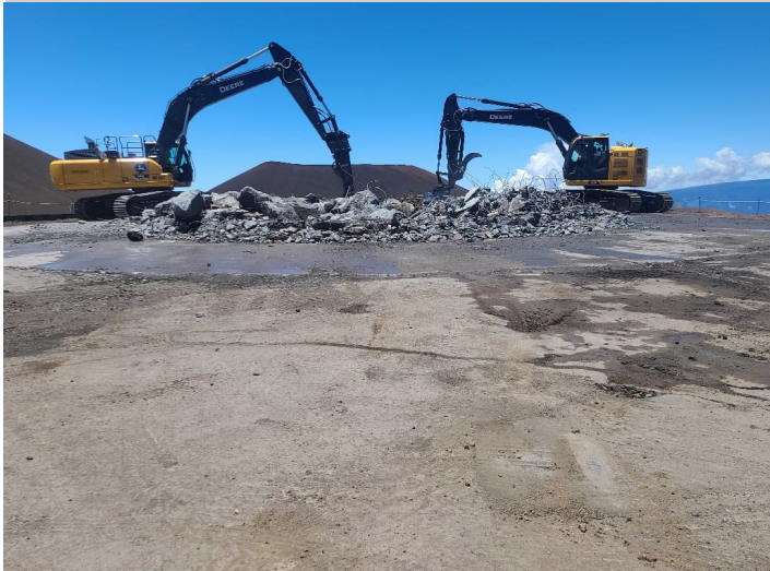
^ Demolition of CSO Reinforced Concrete Foundation
