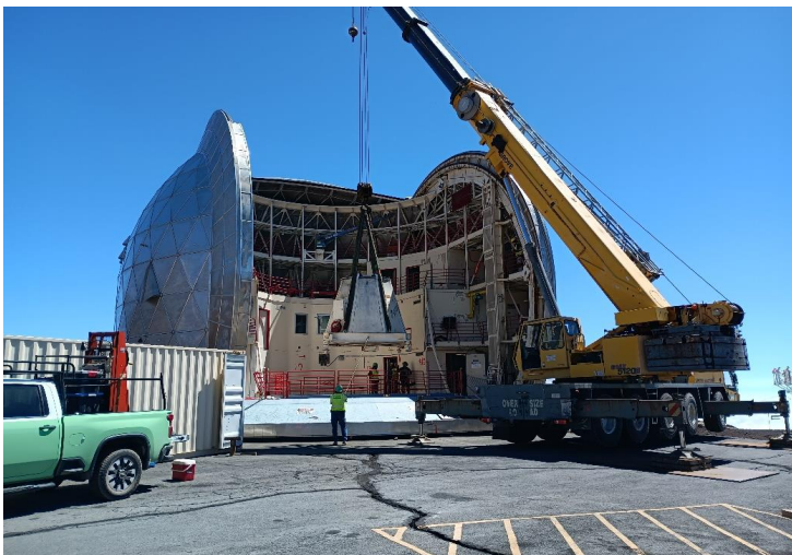
^ 1:57pm - base assy lifted from foundation
