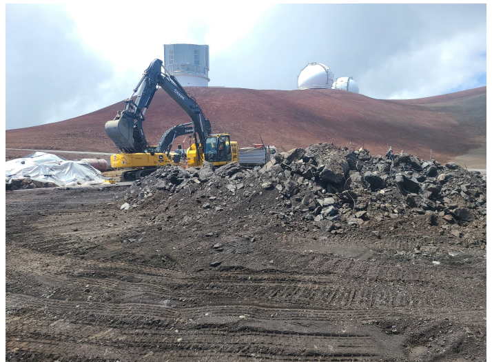
^ CSO Concrete Apron Demolition and Stockpile
