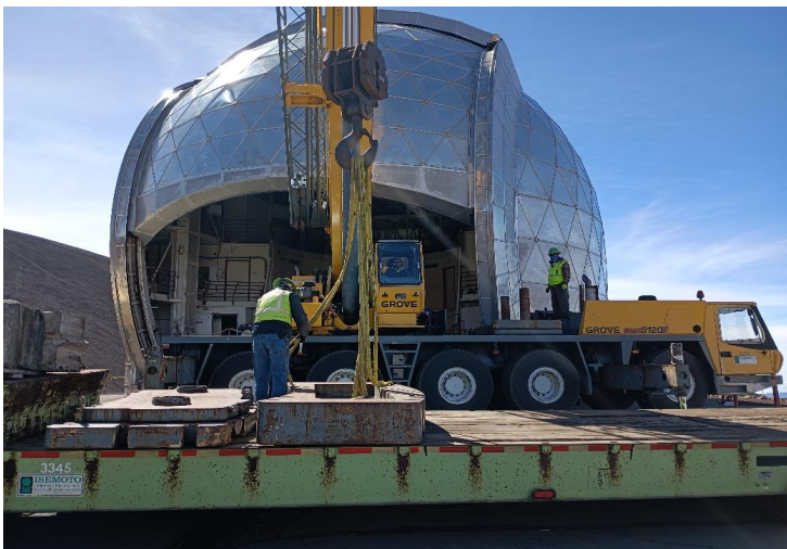
^ 9:30am - loading counterweights on lowboy
