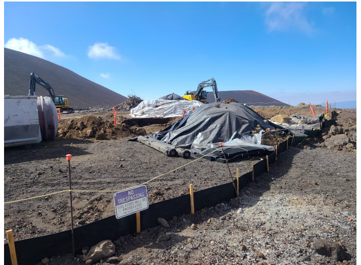
^ Covered Stockpiles of Cesspool Soils Pending Test Results
