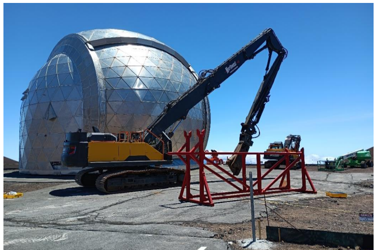
^ 1:09pm - shears attachment installed
