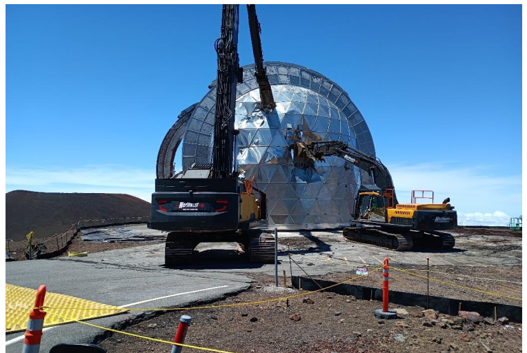
^ 11:19am - punching the side wall into the dome
