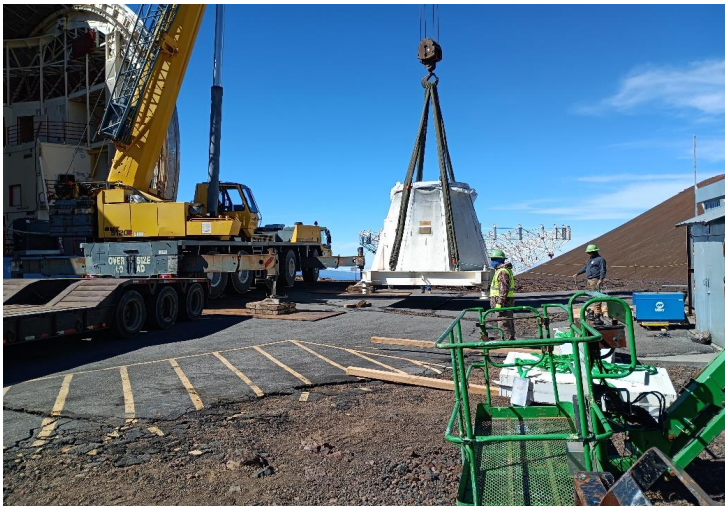
^ 9:30am - picking base assy from ground
