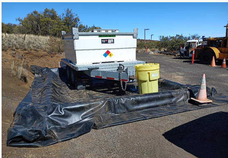
^ 3:11pm - fuel trailer in secondary containment
