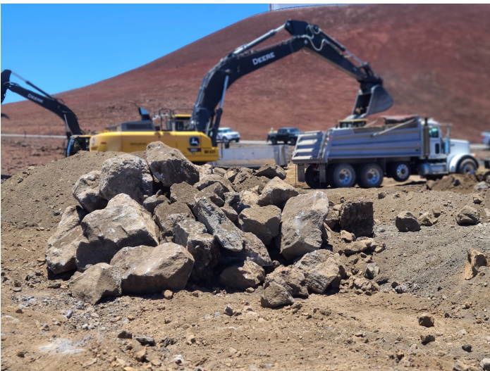
^ Loading Clean Stone for Haul to Batch Plant Area
