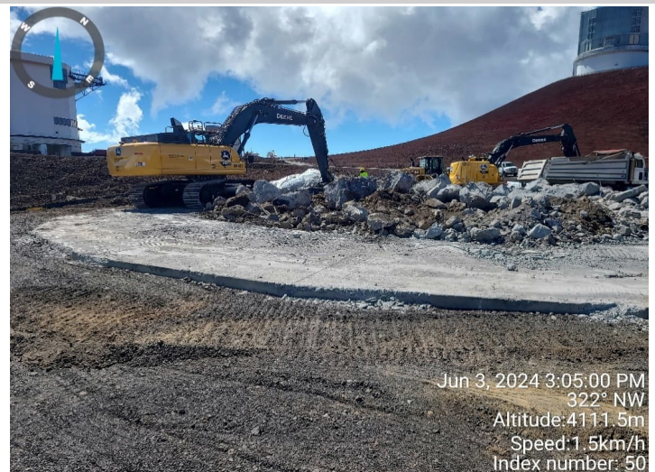
^ Demolition of CSO Reinforced Concrete Foundation
