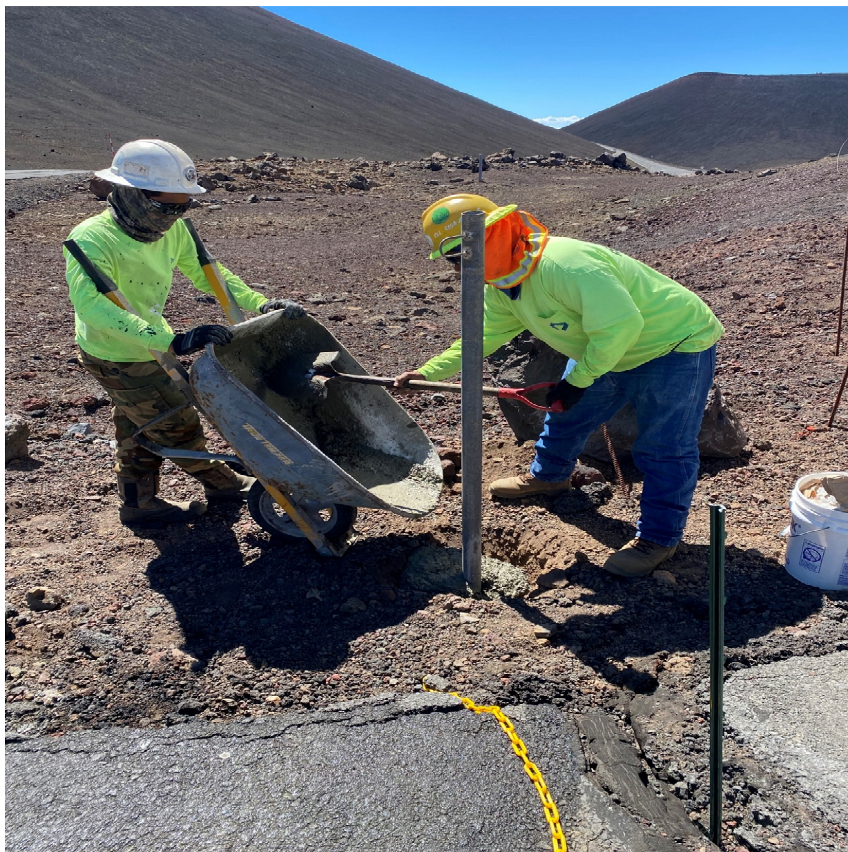
Fence Post Installation
