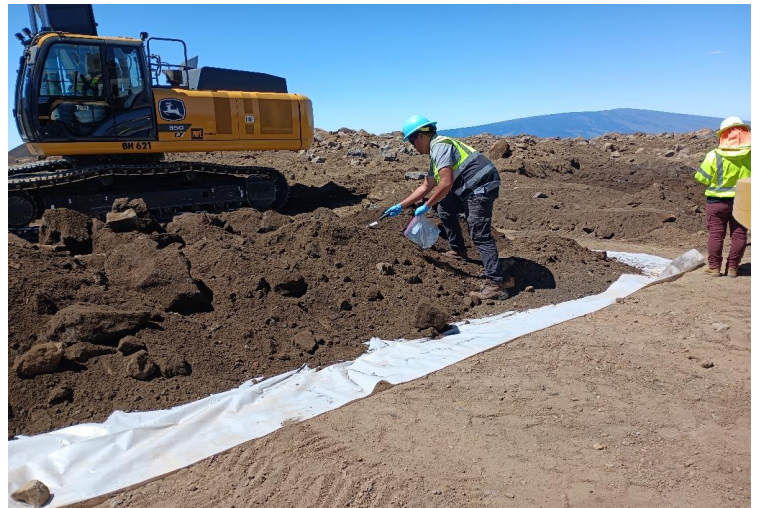
^ 10:29am - sampling excavated material
