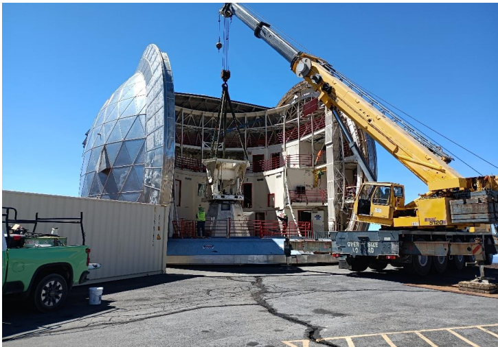
^ 10:24am - elevation assy separated from base
