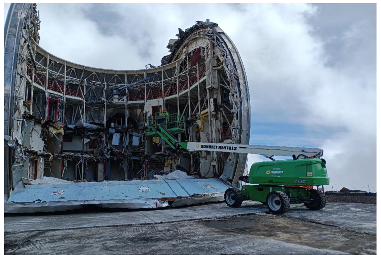
^ 2:10pm - shutter cylinder prepped for removal
