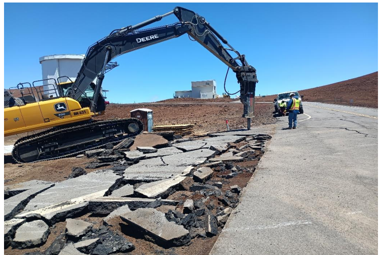
^ 11:26am - demoing asphalt with breaker
