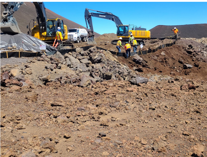
^ Restoring Slope and Silt Fence at Cesspool
