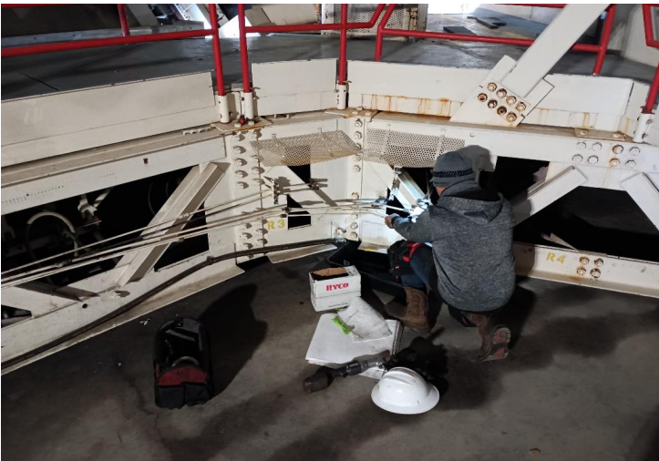
^ 9:15am - removing hydraulic lines
