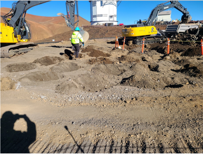
^ Loading Concrete Rubble & Potholing for Soil Sampling
