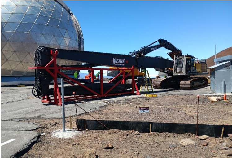
^ 10:46am - excavator connected to boom
