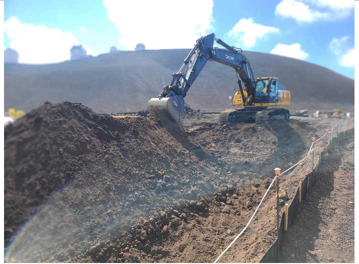
^ Stripping Clean Soil for Haul to Lower CMS Quarry
