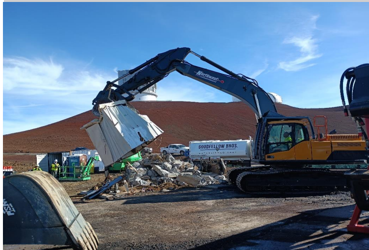
^ 8:07am - demolishing the water shed
