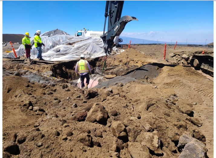
^ Underground Water Tank Excavation
