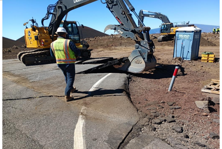
^ 9:46am - starting asphalt demo
