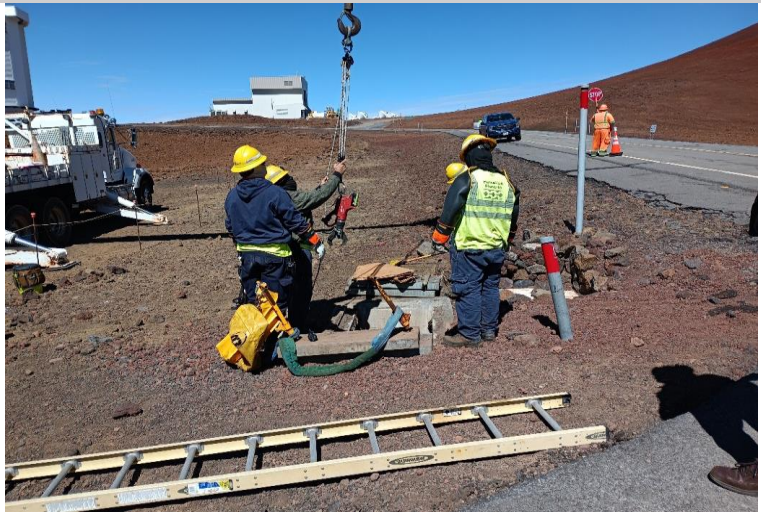
^ 10:57am - prepping to cut cables at pullbox
