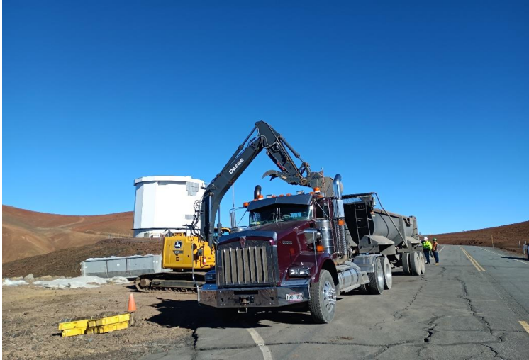
^ 8:00am - loading asphalt debris
