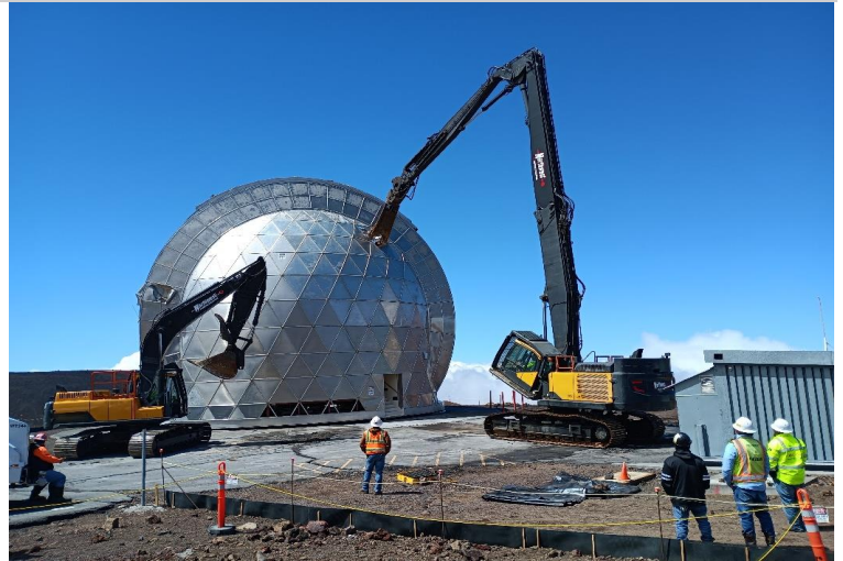
^ 10:26am - removal of aluminum shell begins
