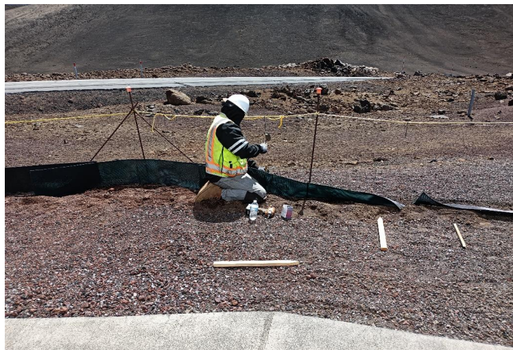
^ 10:18am - installing silt fence
