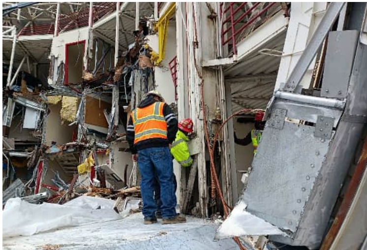
^ 1:15pm - removing bolts from bottom of cylinder
