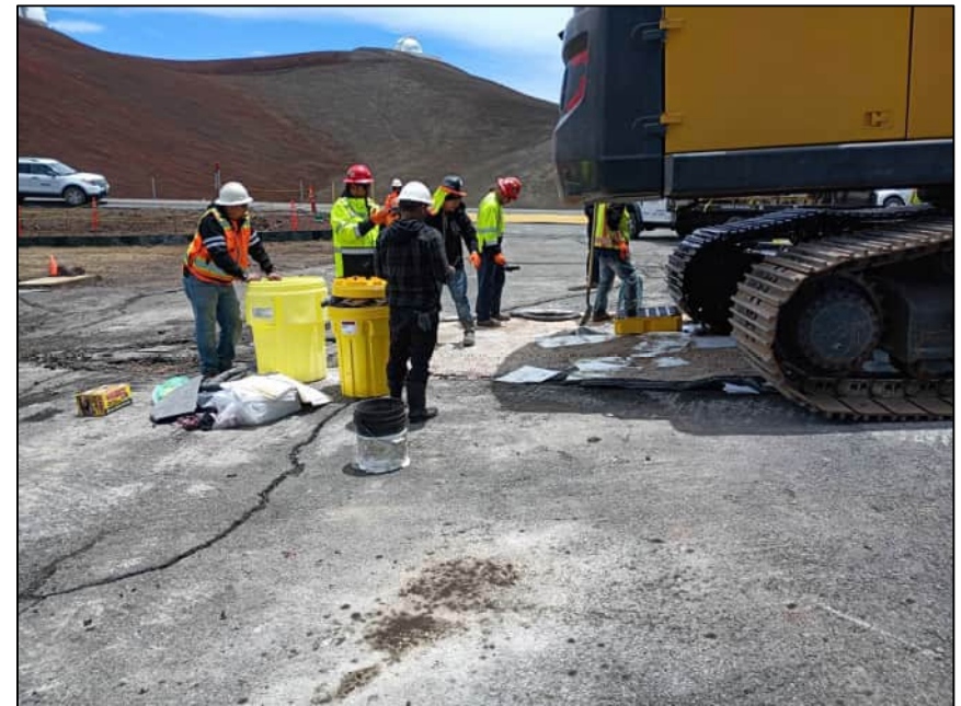
Containerizing and Disposal of Clean Up Material on 4/29/2024
