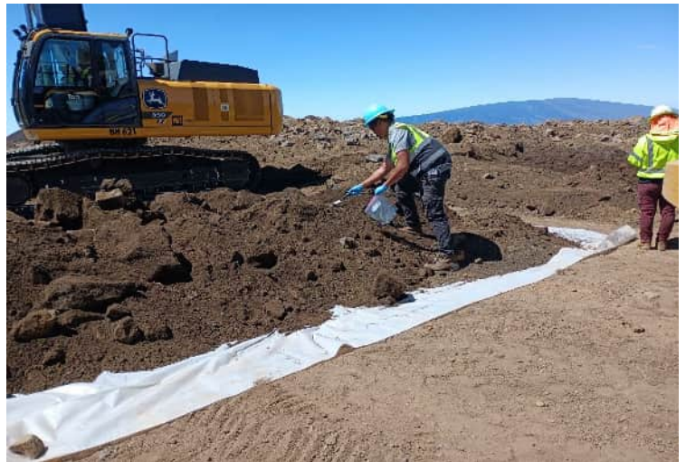
^ 10:29am - sampling excavated material
