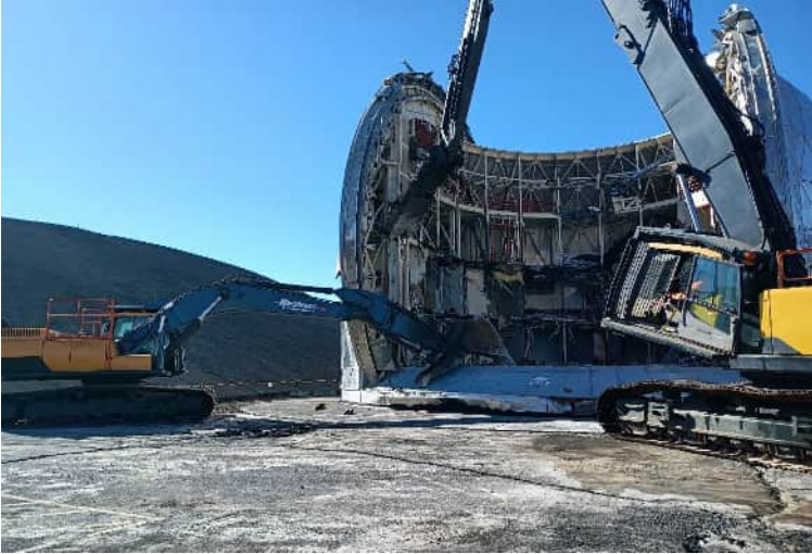
^ 8:25am - housing demo for cylinder removal
