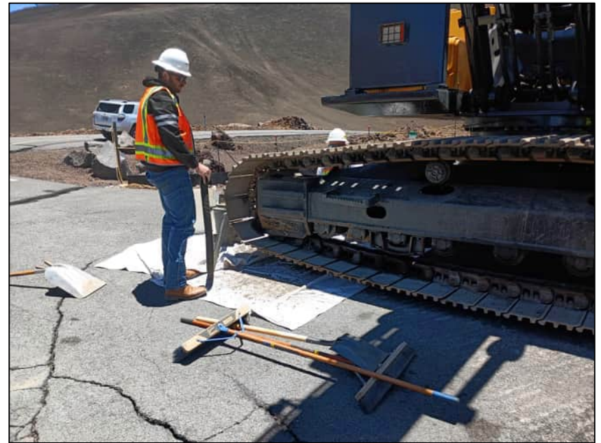
Crew Scrapes Dried Mud on Plastic Sheetting for Proper Disposal
