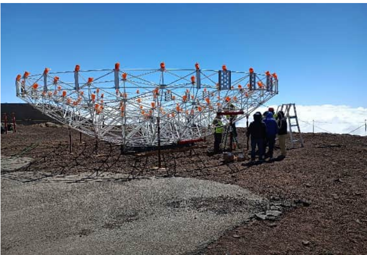
^ 1:26pm - work on BUS disassembly
