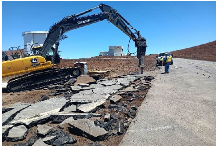
^ 11:26am - demoing asphalt with breaker
