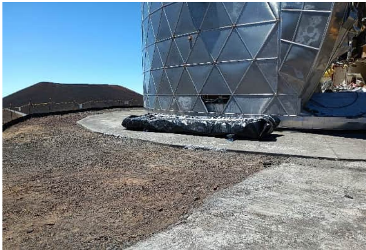
^ 11:17pm - cylinders double wrapped, awaiting transport from site
