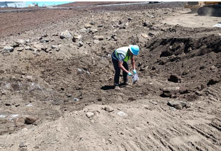
^ 10:49am - sampling in excavation
