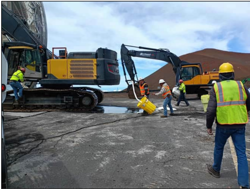
Absorbent Socks from Spill Kit Deployed on 4/30/2024 to Clean up Oil Spill
