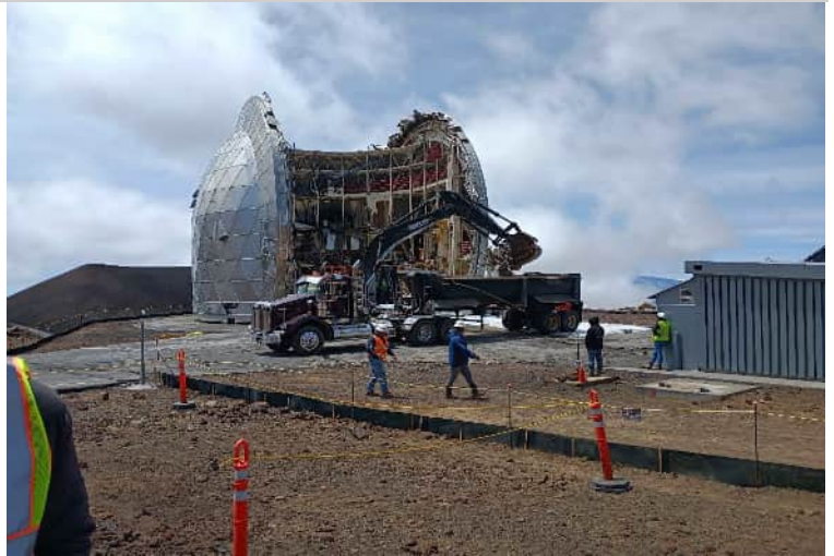
^ 11:17am - loading last truck
