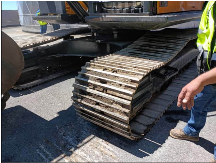
Dried Mud in Excavator Tracks Upon Arrival to the Site
