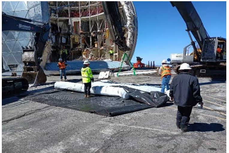
^ 10:06am - removing second cylinder, first is wrapped
