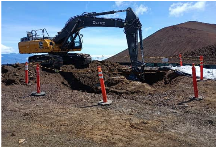
^ 2:38pm - cesspool excavation cordoned off
