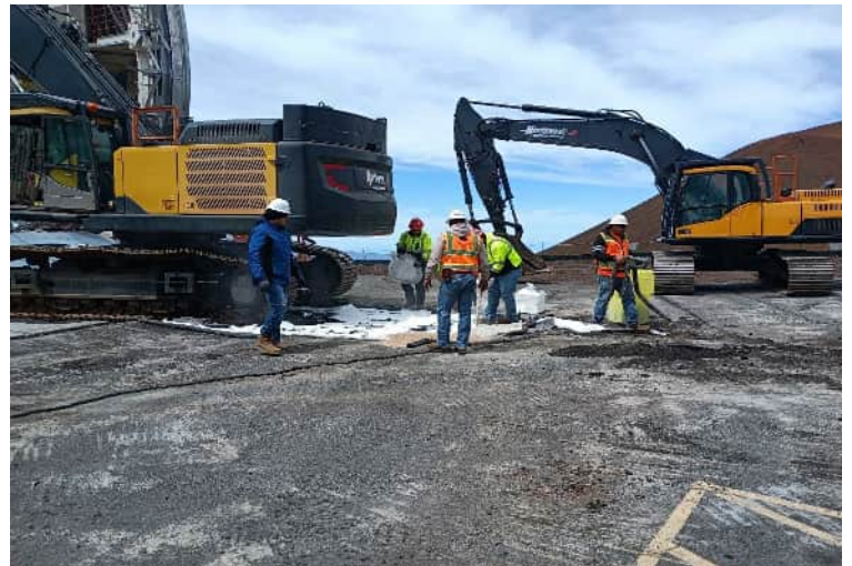
^ 10:35:46am - perimeter contained and materials being placed
