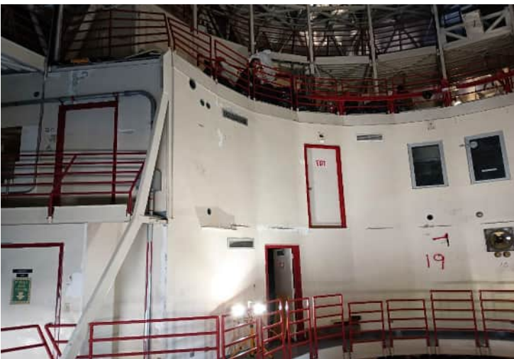
^ 12:47pm - demo progress on 3rd level
