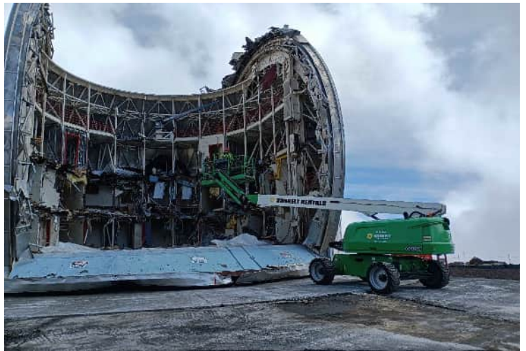
^ 2:10pm - shutter cylinder prepped for removal
