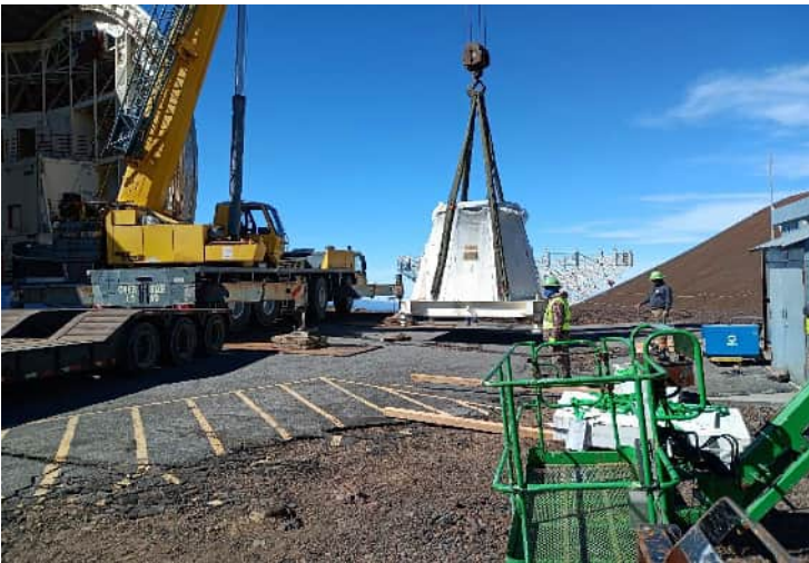
^ 9:30am - picking base assy from ground
