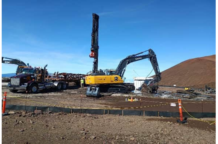
^ 9:07am - breaking outbuilding foundation
