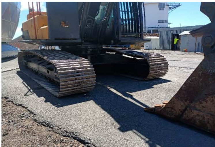
^ 2:05pm - track cleaning completed
