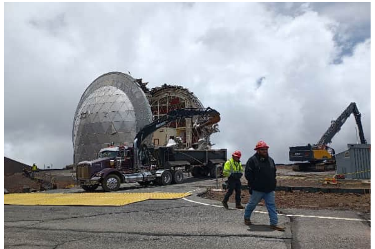
^ 12:36pm - loading demoed material
