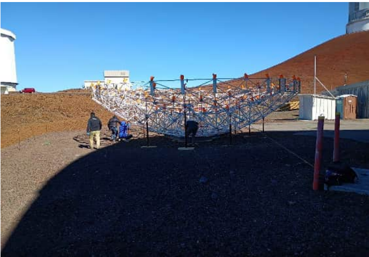
^ 8:55am - working on BUS disassembly
