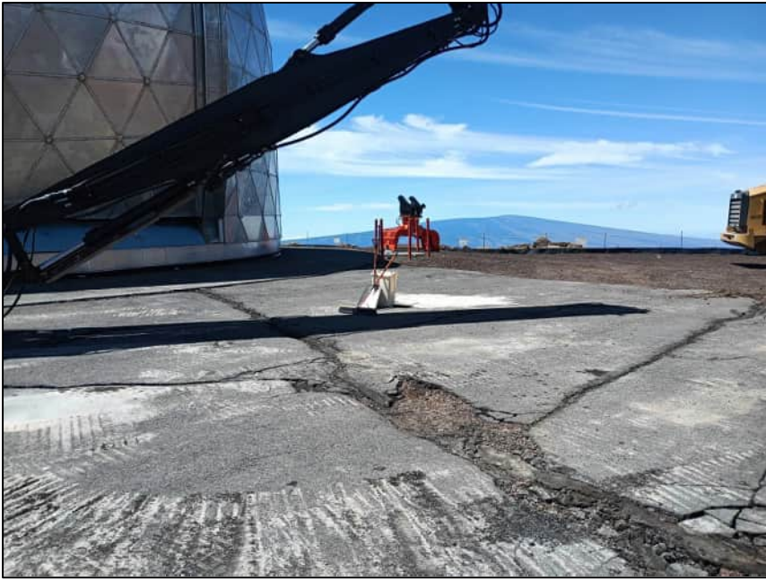
General View of Ground Condition Following Clean Up
