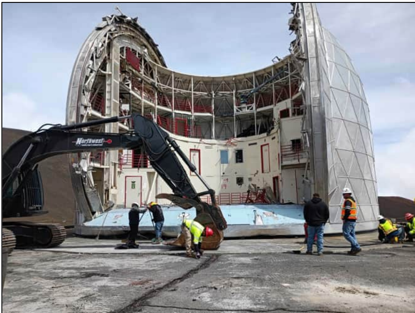
Excavator Oil Leak Clean Up in Progress on 4/29/2024
