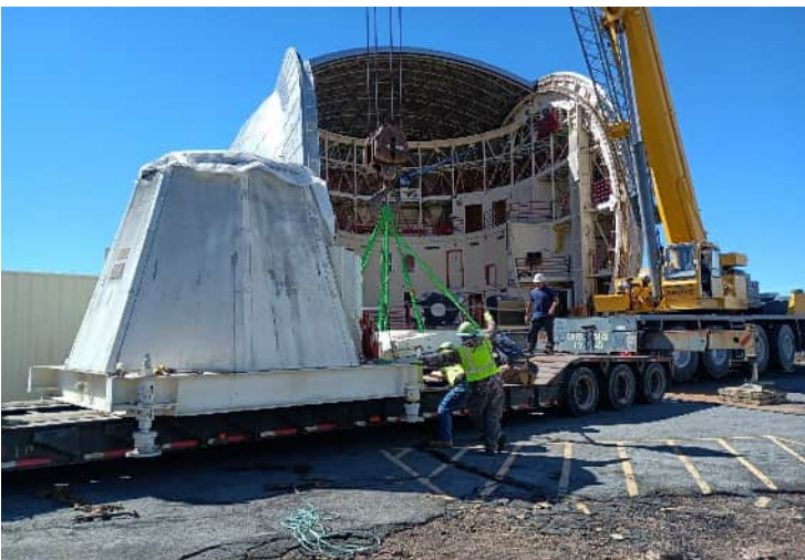
^ 9:45am - counterweight positioned on lowboy
