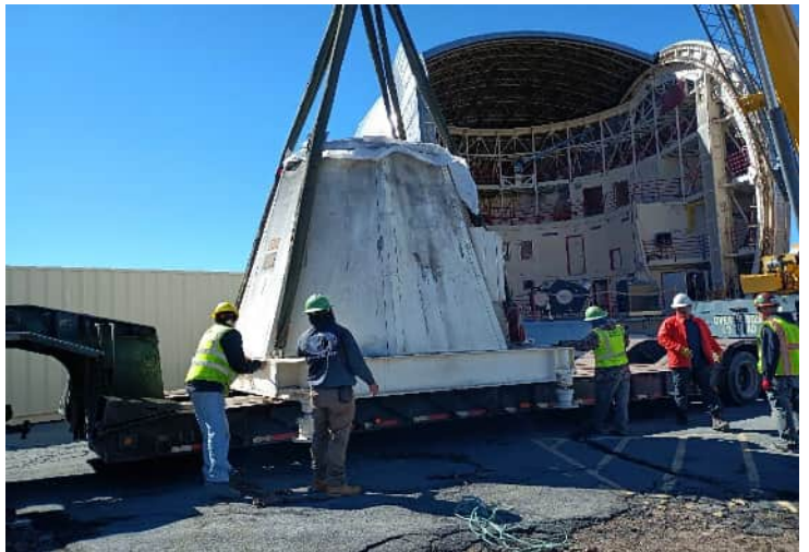
^ 9:33am - base assy positioned on lowboy
