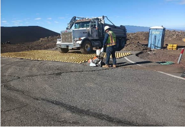
^ 8:18am - sawcutting pavement
