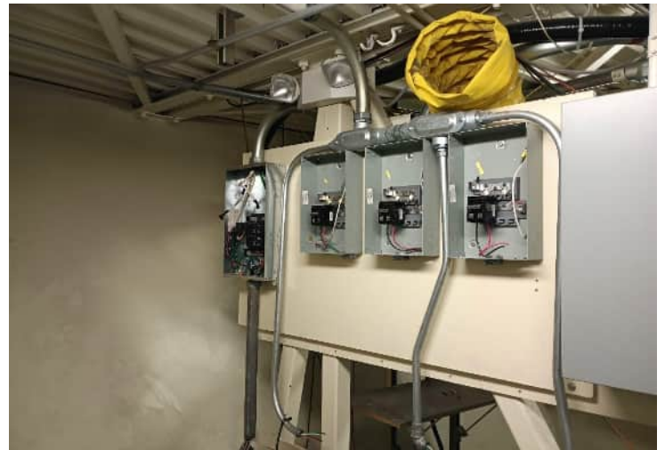
^ 12:44pm - progress in electric room
