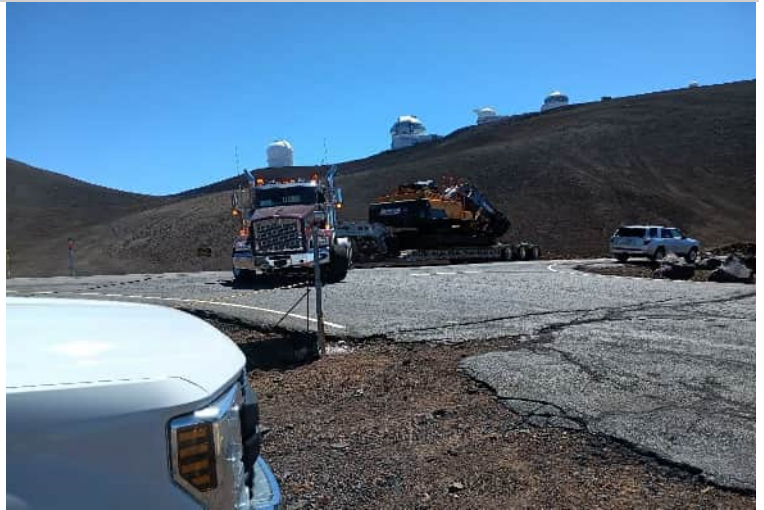
^ 10:29am - excavator arrives at site
