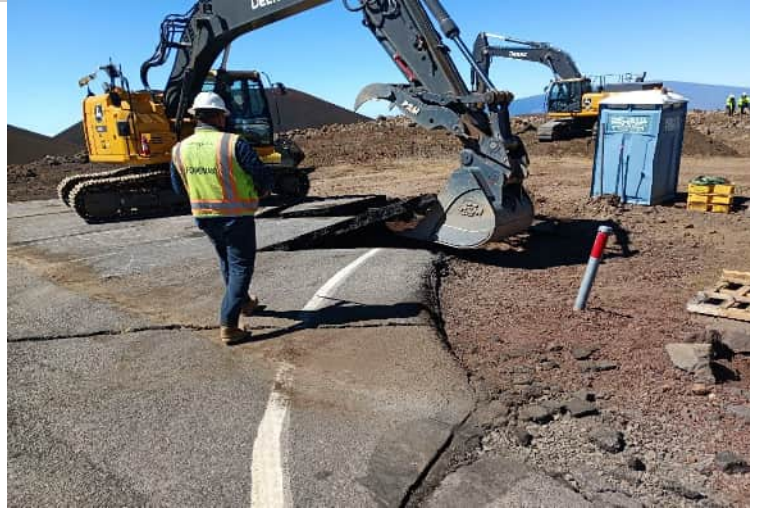
^ 9:46am - starting asphalt demo
