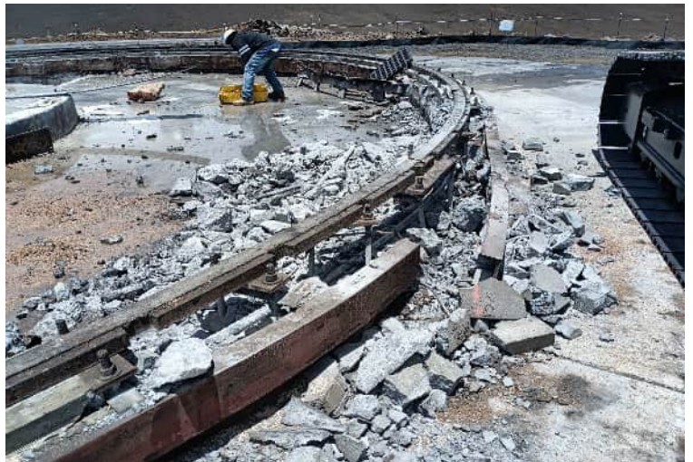
^ 12:52pm - demolded section of rail ring (dust control water visible)
