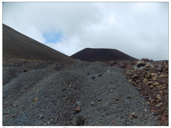
Figure 20. Recently dumped cinder fill in staging area, view to the east.
