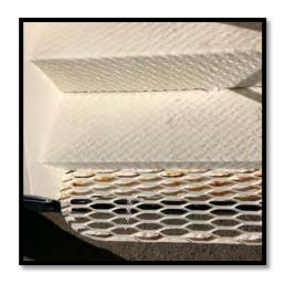
L-5: (5,200 mg/kg) Lead-Based Paint
