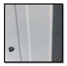
L-15: (69,000 mg/kg) Lead-Based Paint
