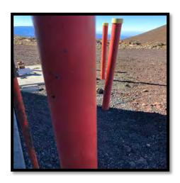
L-1: (150,000 mg/kg) Lead-Based Paint
