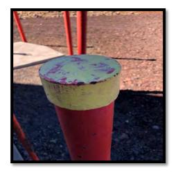
L-2: (140,000 mg/kg) Lead-Based Paint
