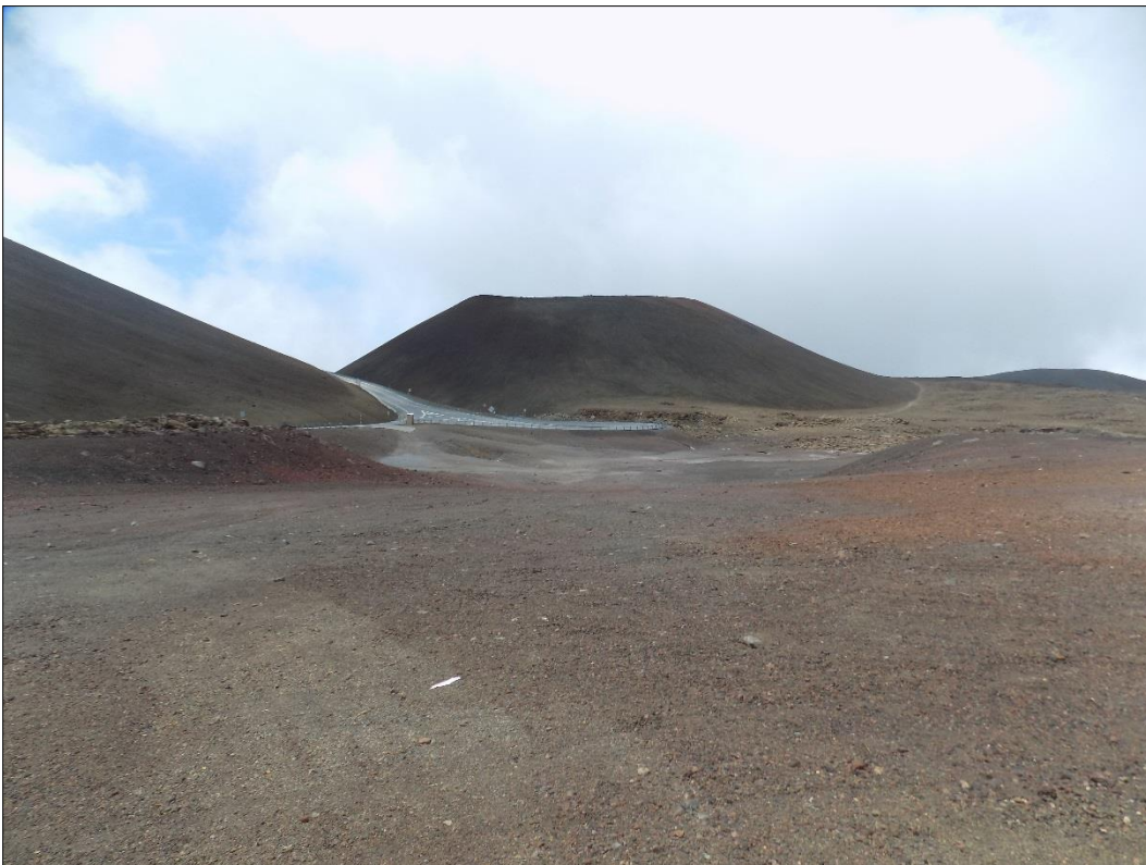
Figure 7. Batch plant area, view to the southeast.
