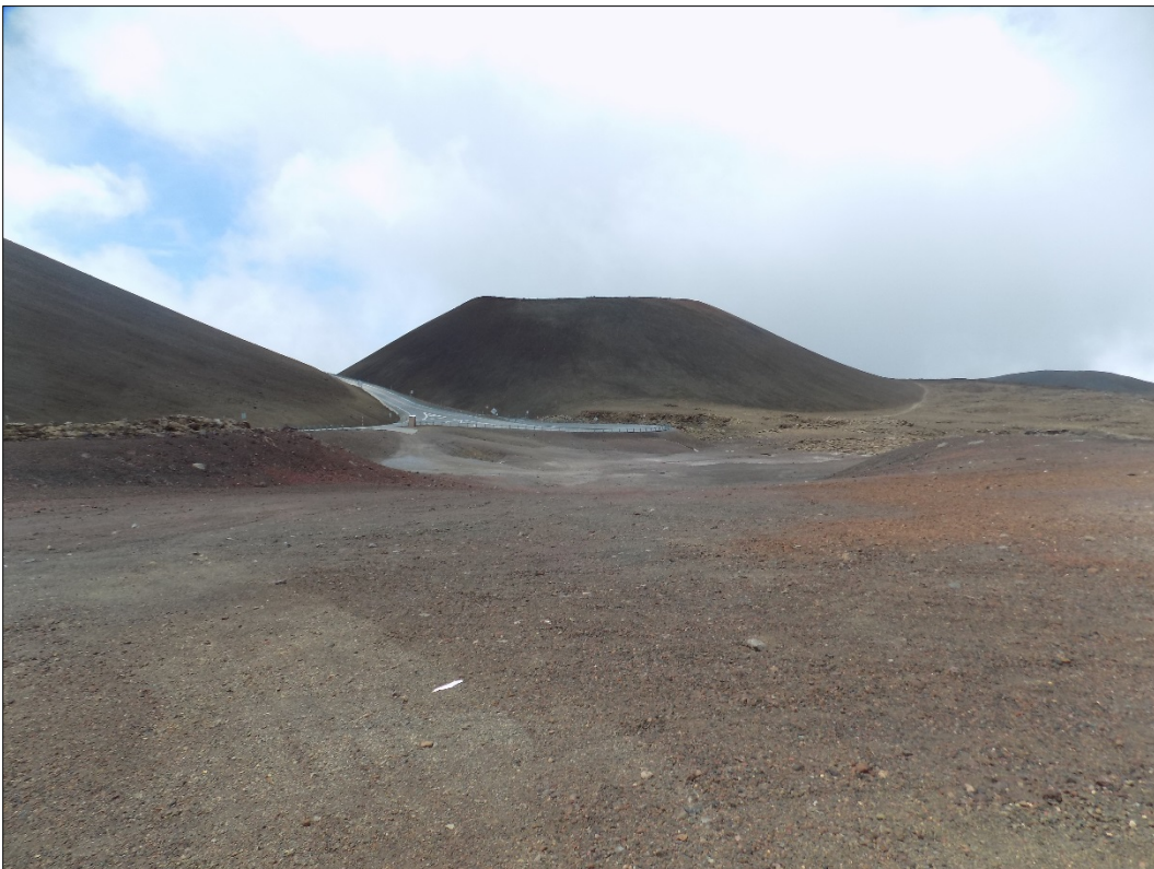
Figure 5. Batch plant area, view to the southeast.
