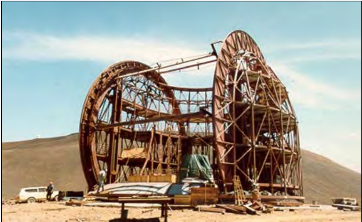
Figure 5-5: CSO's Internal Structure During Construction
