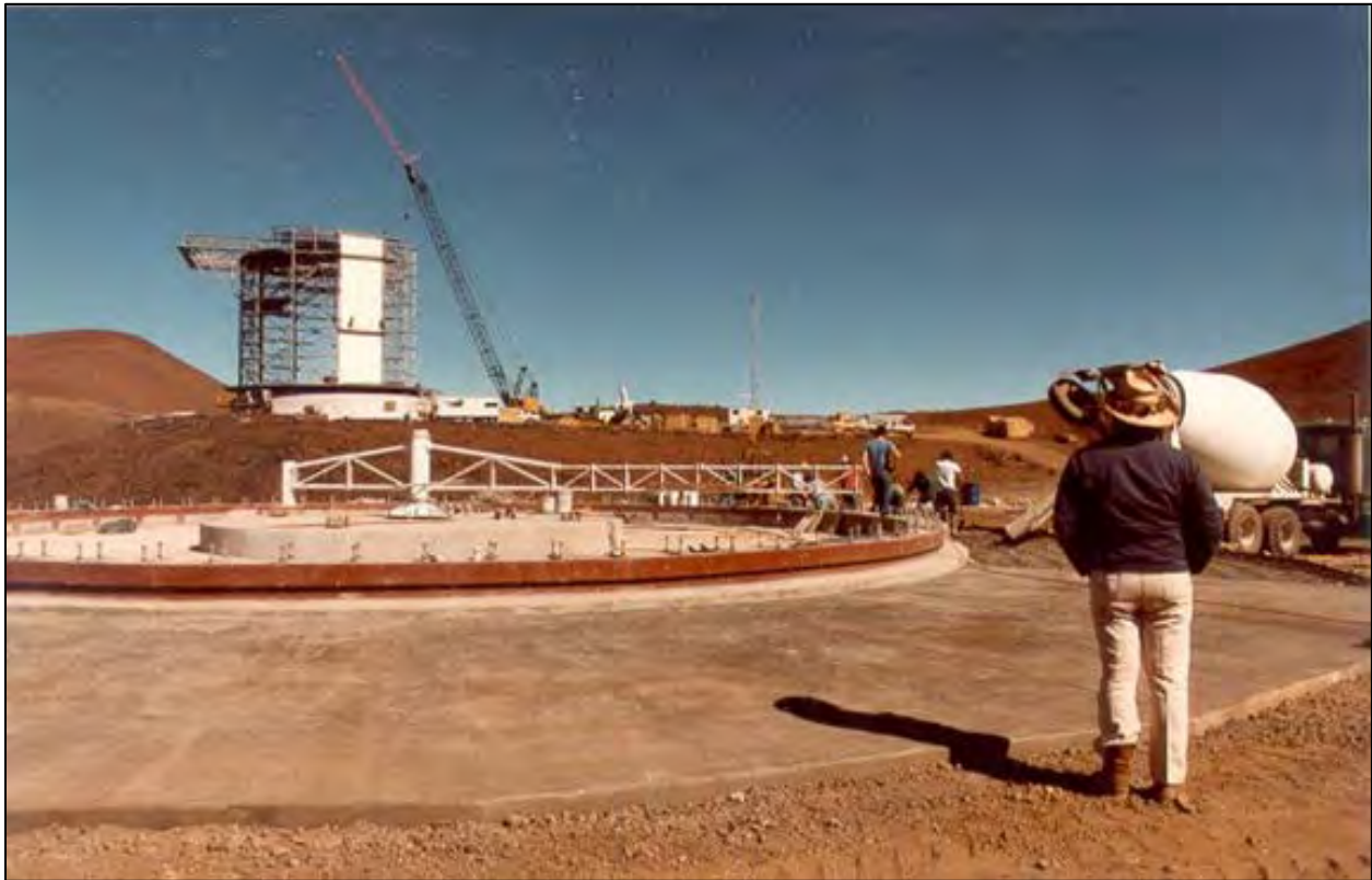
Figure 5-6: Photograph of CSO's Foundation During Construction
