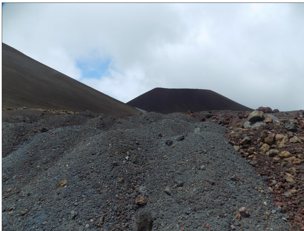
Figure 20. Recently dumped cinder fill in staging area, view to the east.
