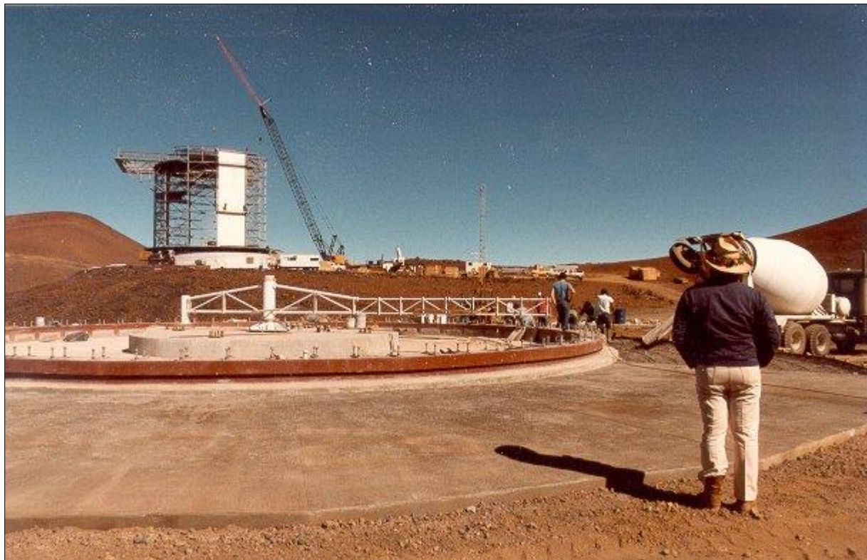
Figure 14. CSO under construction, view to the northwest (Steiger 2009).
