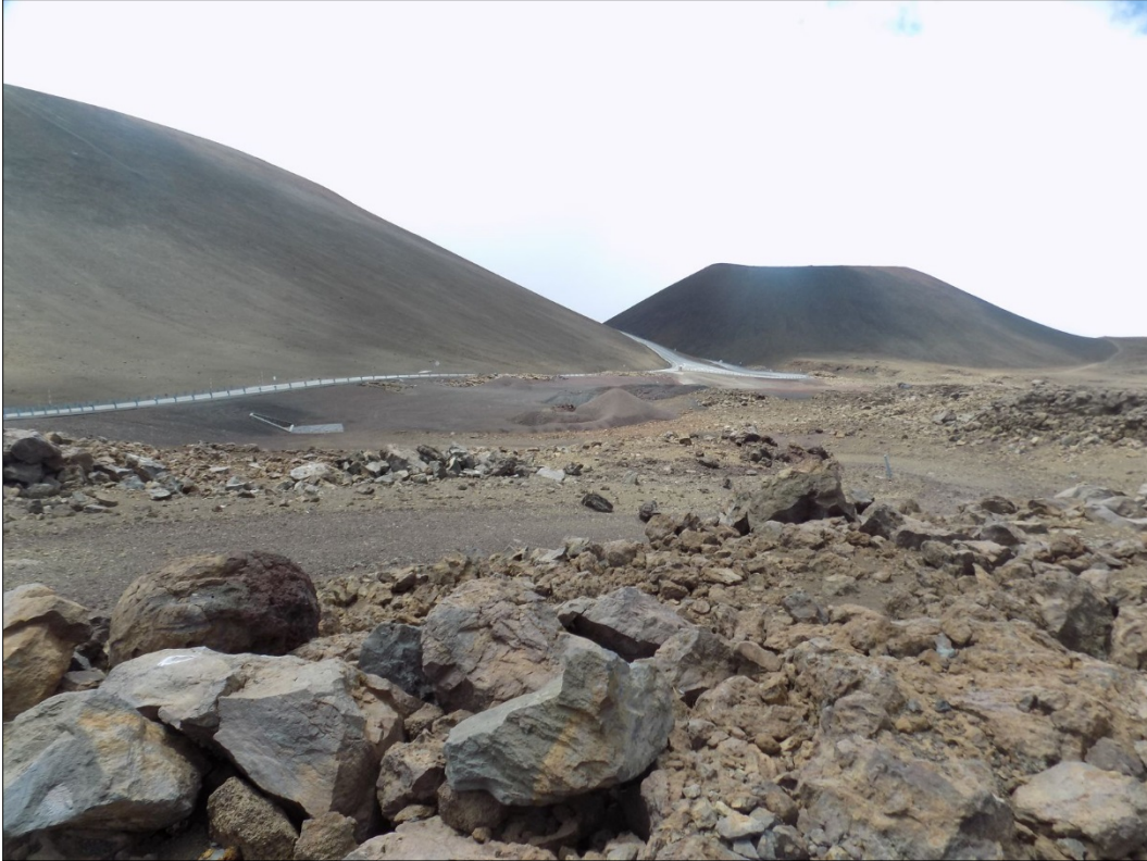
Figure 4. Unpaved access road (foreground) leading to batch plant area, view to the southeast.
