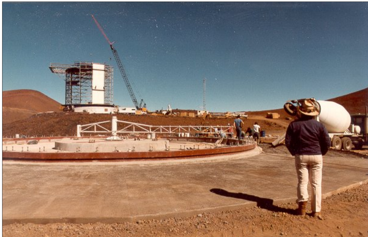
Figure 12. CSO under construction (in foreground), view to the north (Steiger 2009).
